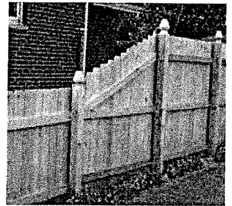
example of acceptable transition from 4' to 6'
