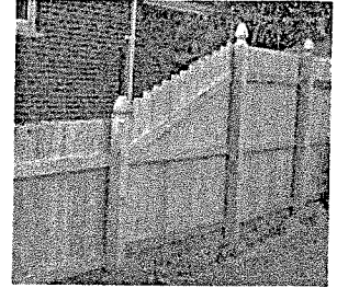
example of acceptable transition from 4' to 6'
